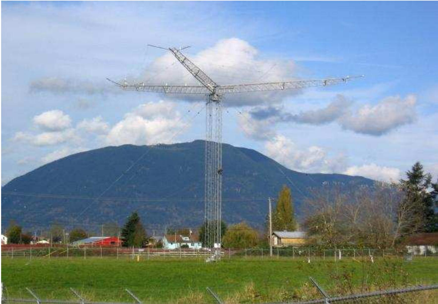
Conical monopole - an omni-directional, medium range HF antenna. There are four of these on site
